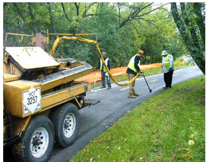
Asphalt crack repair and seal combined
