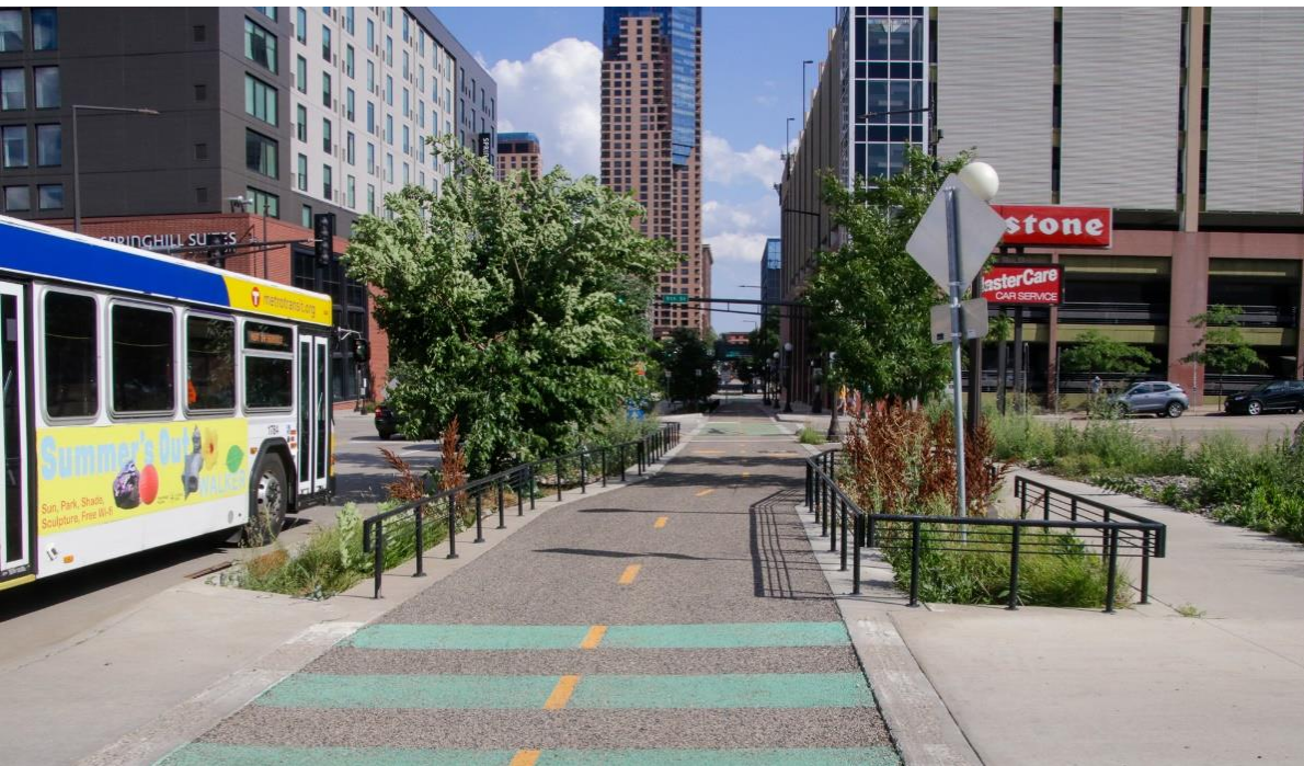
The surface of the Jackson Street (St. Paul, MN) two-way grade-separated bikeway (or two-way cycle track) is a porous asphalt that helps with stormwater management, winter maintenance and rideability. The landscaped buffers are bio-filtration basin and tree trench systems to provide filtration of stormwater runoff and snow storage in the winter.
