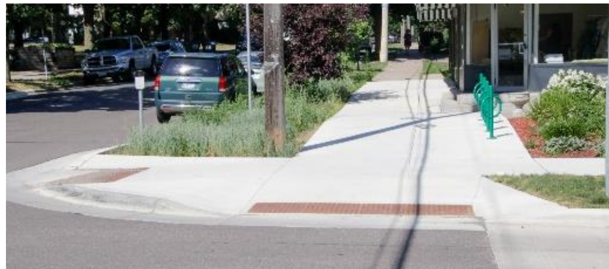
Curb extensions (or bump-outs) provide space for rain gardens, native plants and snow storage while reducing crossing distances for people on foot.
