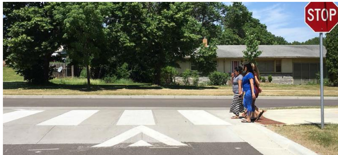
Raised Table crosswalks work well at side streets or driveways to give people walking or biking priority, reinforce motorist stop location, slow motorist turning speeds and increase motorist yielding behavior.
