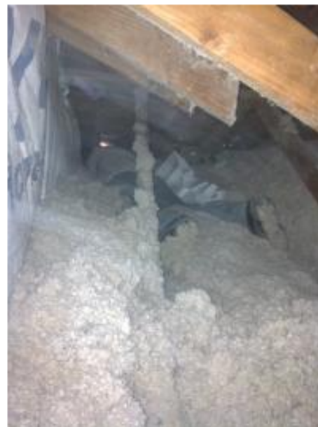
Climbing through insulation in attic.
